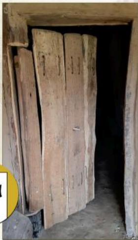
2019: Reconstructed doors at the Pennigbüttel house
