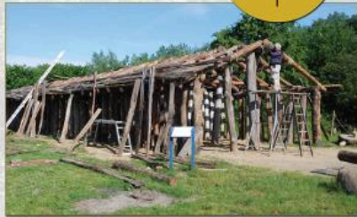
2019: After about 20 years we rebuilt the house. The roof partially collapsed at the rear of the house. When we tried to make it secure for the public again we learned that we needed to rebuild it completely.
