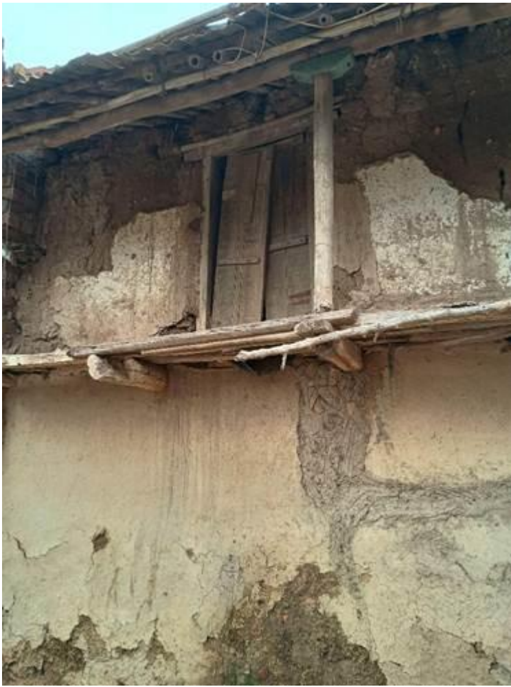
FIG 4. A MUD HOUSE WITH A BROKEN WOODEN PROJECTING BALCONY. PHOTO BY ANSHIKA SINGH (2025)
