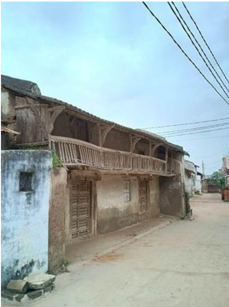
FIG 4. A MUD HOUSE WITH A BROKEN WOODEN PROJECTING BALCONY. PHOTO BY ANSHIKA SINGH (2025)
