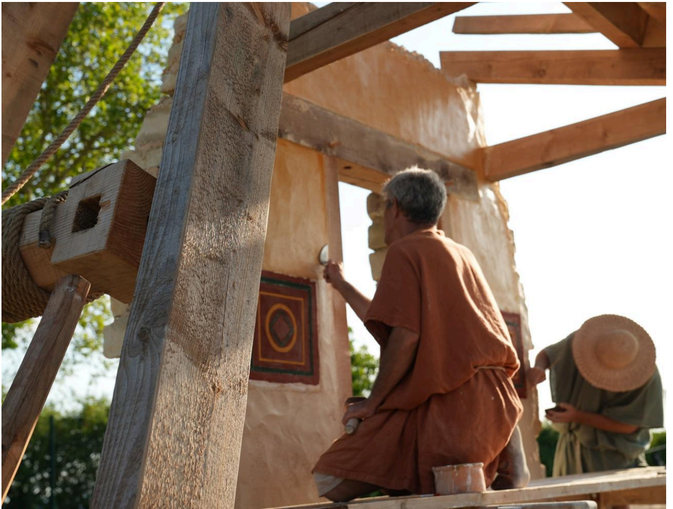
FIG 7. THE PAINTER SMOOTHES THE SURFACE OF THE FINAL PLASTER COAT, TO COVER UP THE WOODEN FRAME OF THE PAINTED PINAKES. PHOTO BY ALEXANDRE BOULOUMOU.
