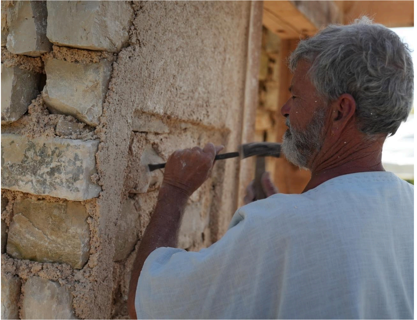
FIG 5. THE MASON IS REMOVING PROTRUDING PARTS OF THE STONES, SO THAT THE PAINTINGS CAN BE INSERTED CORRECTLY. PHOTO BY ALEXANDRE BOULOUMOU.
