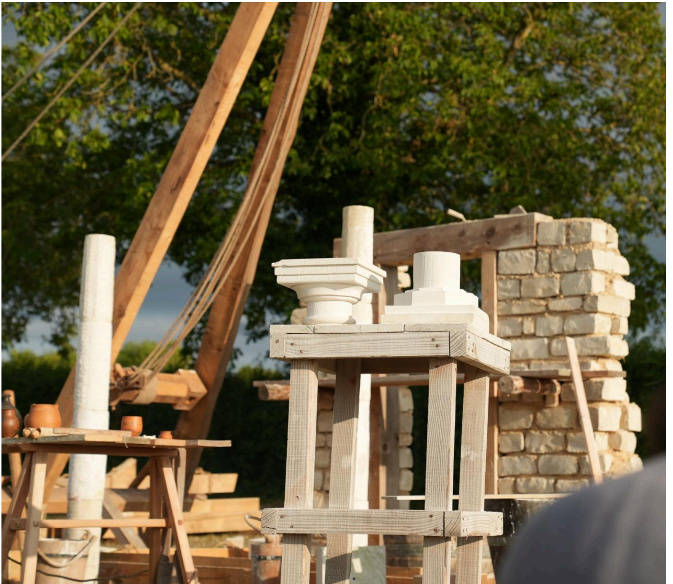
FIG 2. THE TWO CAPITALS BEING MADE BY THE STONECUTTER, WITH THE PORTICO ENTRYWAY IN THE BACK. PHOTO BY ALEXANDRE BOULOUMOU.
