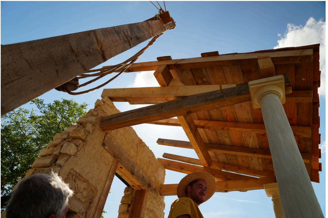
FIG 3. THE COMPLETE TIMBER FRAME, SITTING ON TOP OF THE COLUMNS AND THE FINISHED WALL. PHOTO BY ALEXANDRE BOULOUMOU.
