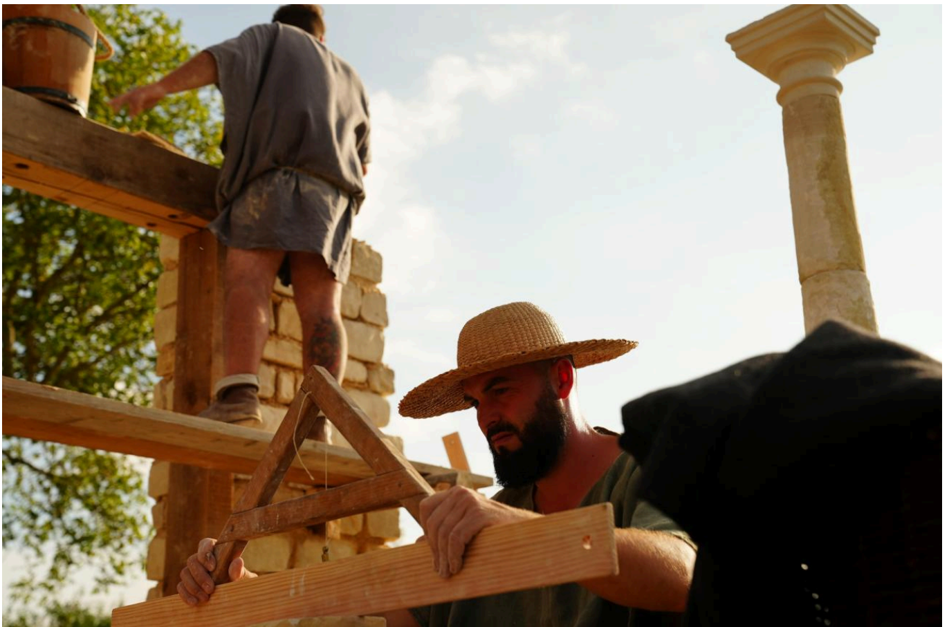
FIG 1. THE LIBELLA BEING USED TO CHECK THE HORIZONTALITY OF THE GROUND ON WHICH COLUMNS ARE BUILT. PHOTO BY ALEXANDRE BOULOUMOU.
