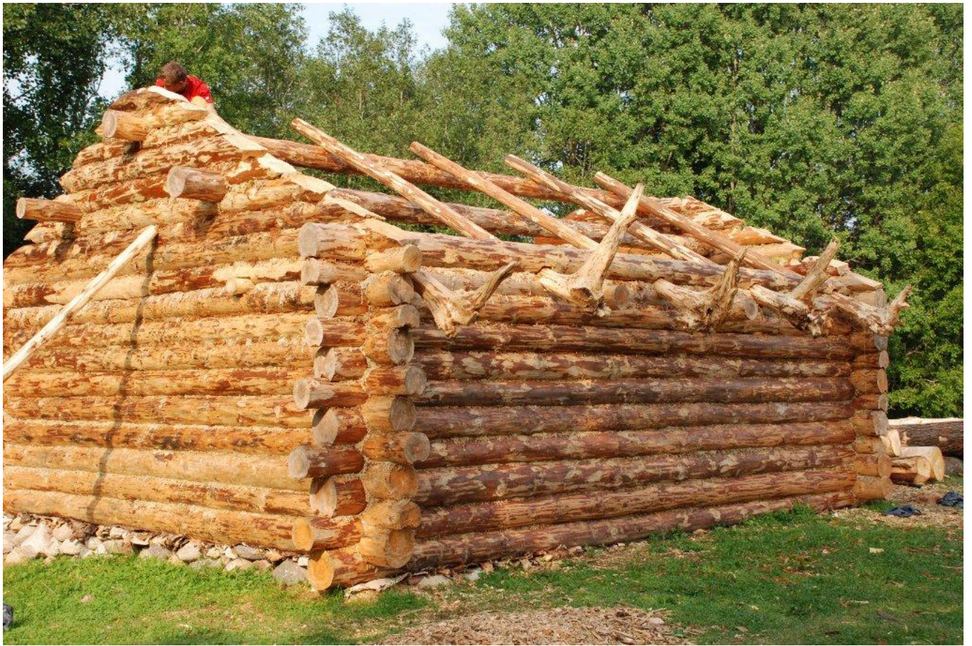
FIG 1. THE WALLS ARE FINISHED, THE ROOF CONSTRUCTION IS VISIBLE.
