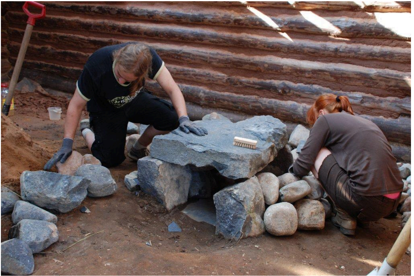
FIG 5. BUILDING THE STOVE. THE BIG PLATE ON TOP HAD TO BE REPLACED, AS IT BROKE IN HALF DURING THE FIRST FIRE.
