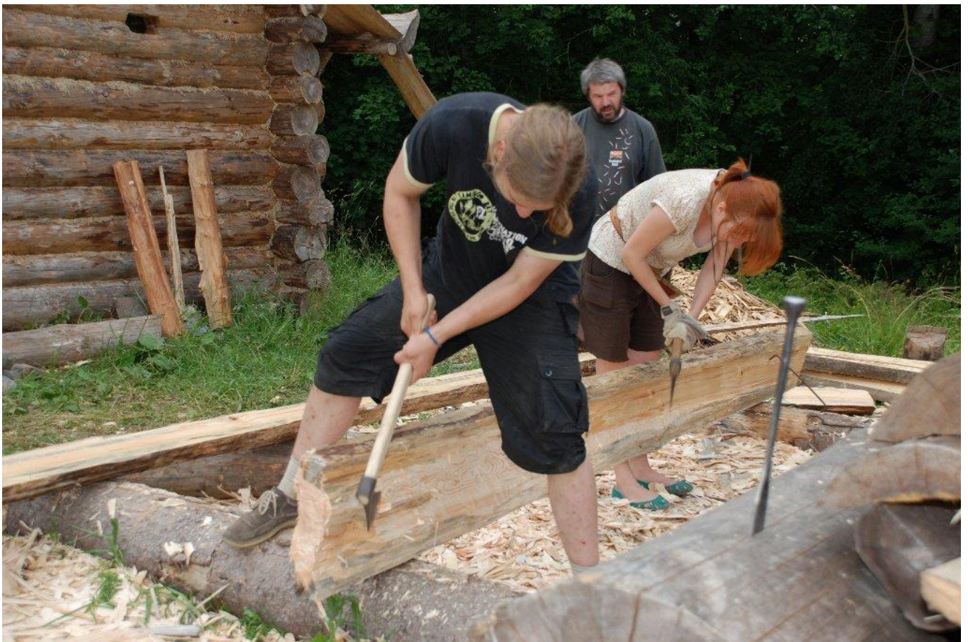
FIG 6. HEWING THE ROOF PLANKS STRAIGHT.
