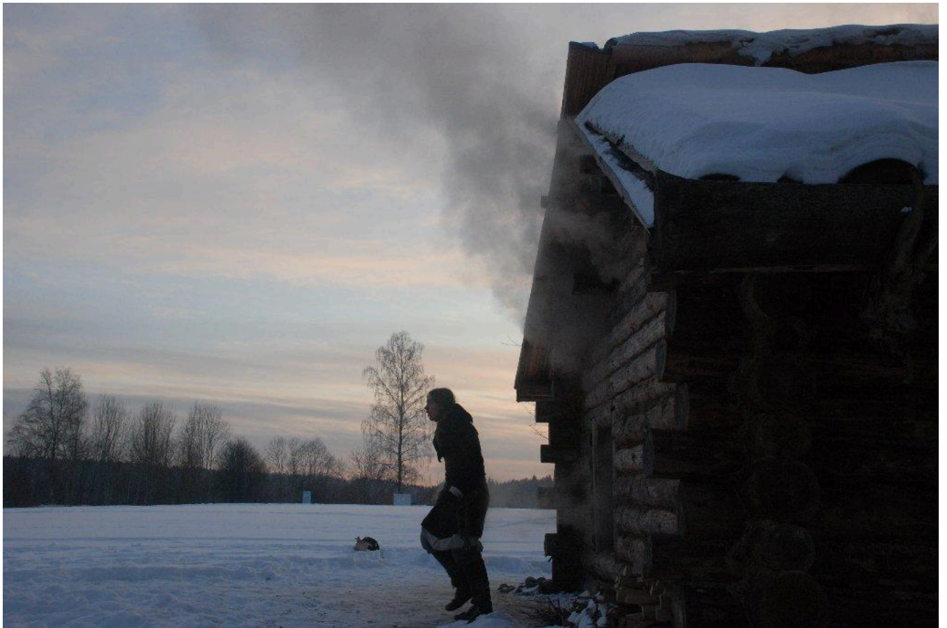
FIG 10. DURING HEATING, THE SMOKE EXITED THROUGH THE DOOR AND MORTISES.
