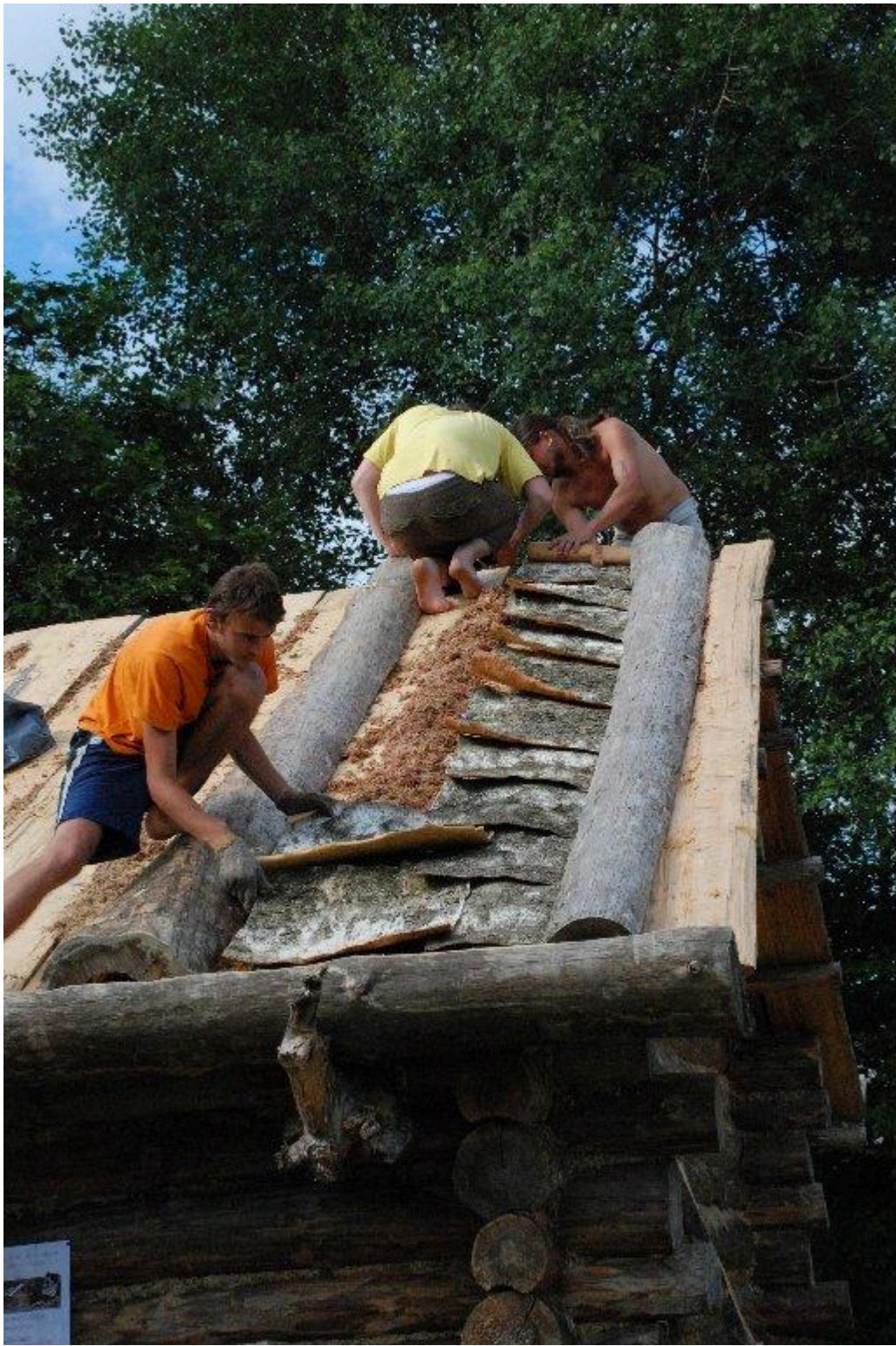
FIG 2. BETWEEN THE ROOF PLANKS, BIRCH BARK AND MOSS WAS PUT.
