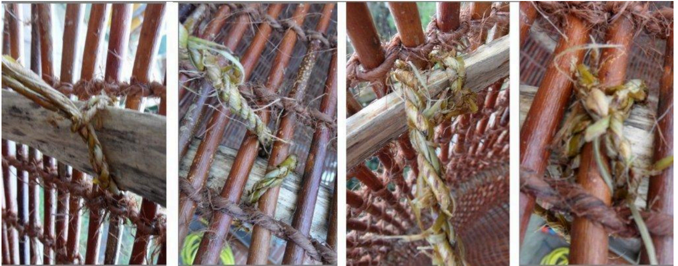
FIG 38. CROSS-STICH LASHING, PHOTO EVA IJSVELD
