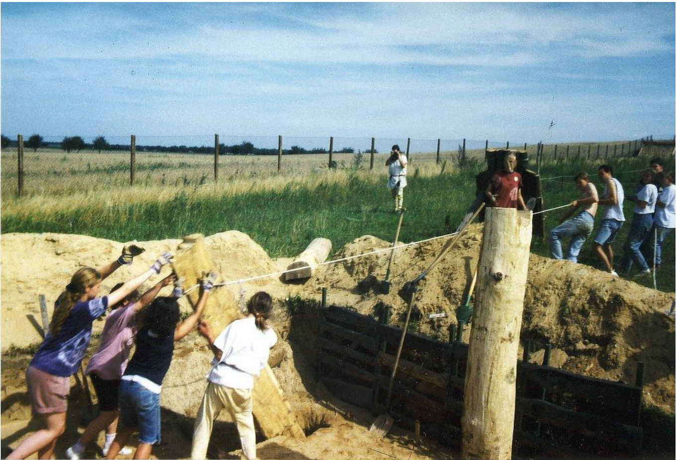
FIG 2. INTERNATIONAL YOUTH WORK CAMP (IJGD) 1993 AT THE LANGOBARDENWERKSTATT ZETHLINGEN. UNDER GUIDANCE OF A CARPENTER, ADOLESCENTS RAISE THE POSTS OF THE HOUSE. PHOTO R. LEINEWEBER.
