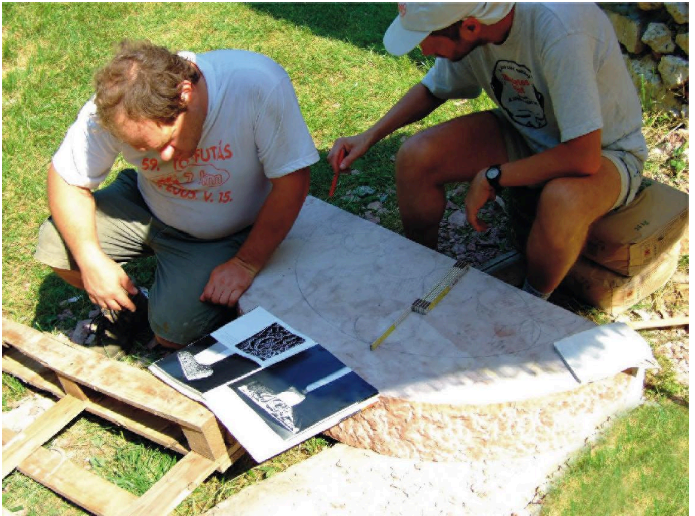
FIG 6A. PICTURES FROM DIFFERENT STAGES OF THE GATE - ARCH RECONSTRUCTION: DRAWING OF THE PATTERN.
