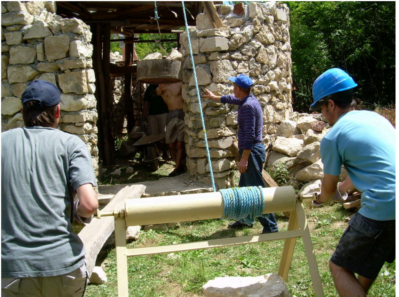
FIG 5C. PICTURES FROM DIFFERENT STAGES OF THE RECONSTRUCTION - STONE LIFTING BY WINDER.
