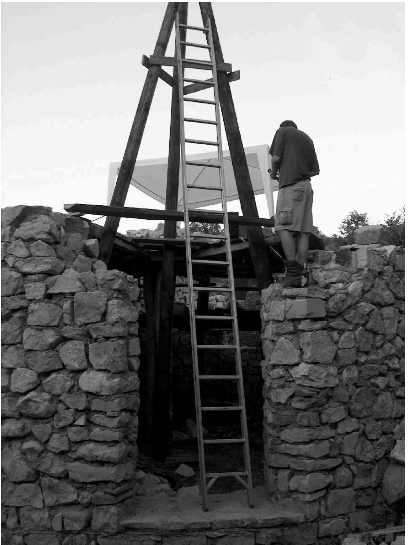
FIG 15A. THE OFTEN HEAVY AND LARGE STONES ARE LIFTED UP TO THE PLATFORM BY HOIST FIXED TO A TRIPOD.
