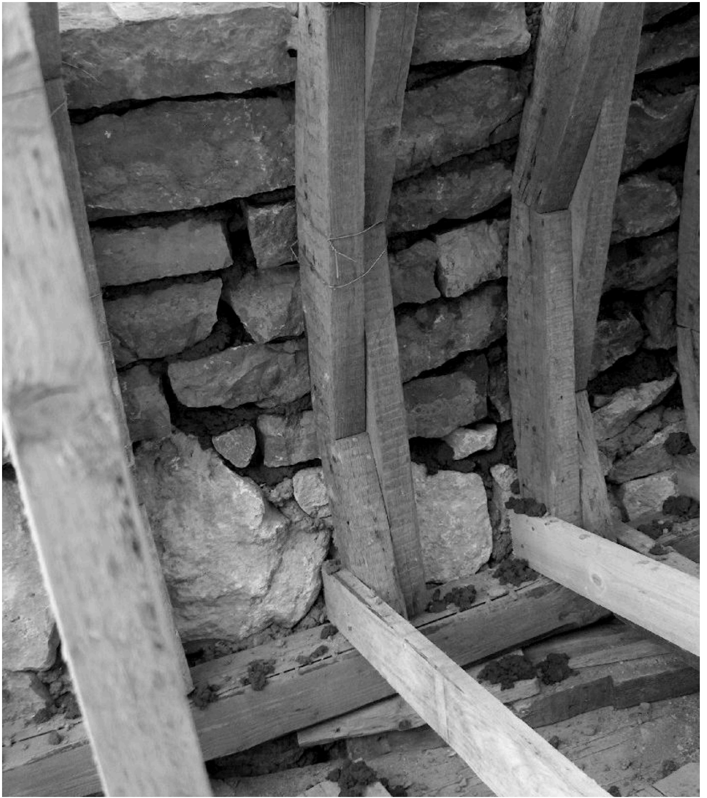
FIG 17A. THE ERECTION OF THE APSE VAULTING - MASTER SHAPES POSITIONED 25-30 CM FROM EACH OTHER.
