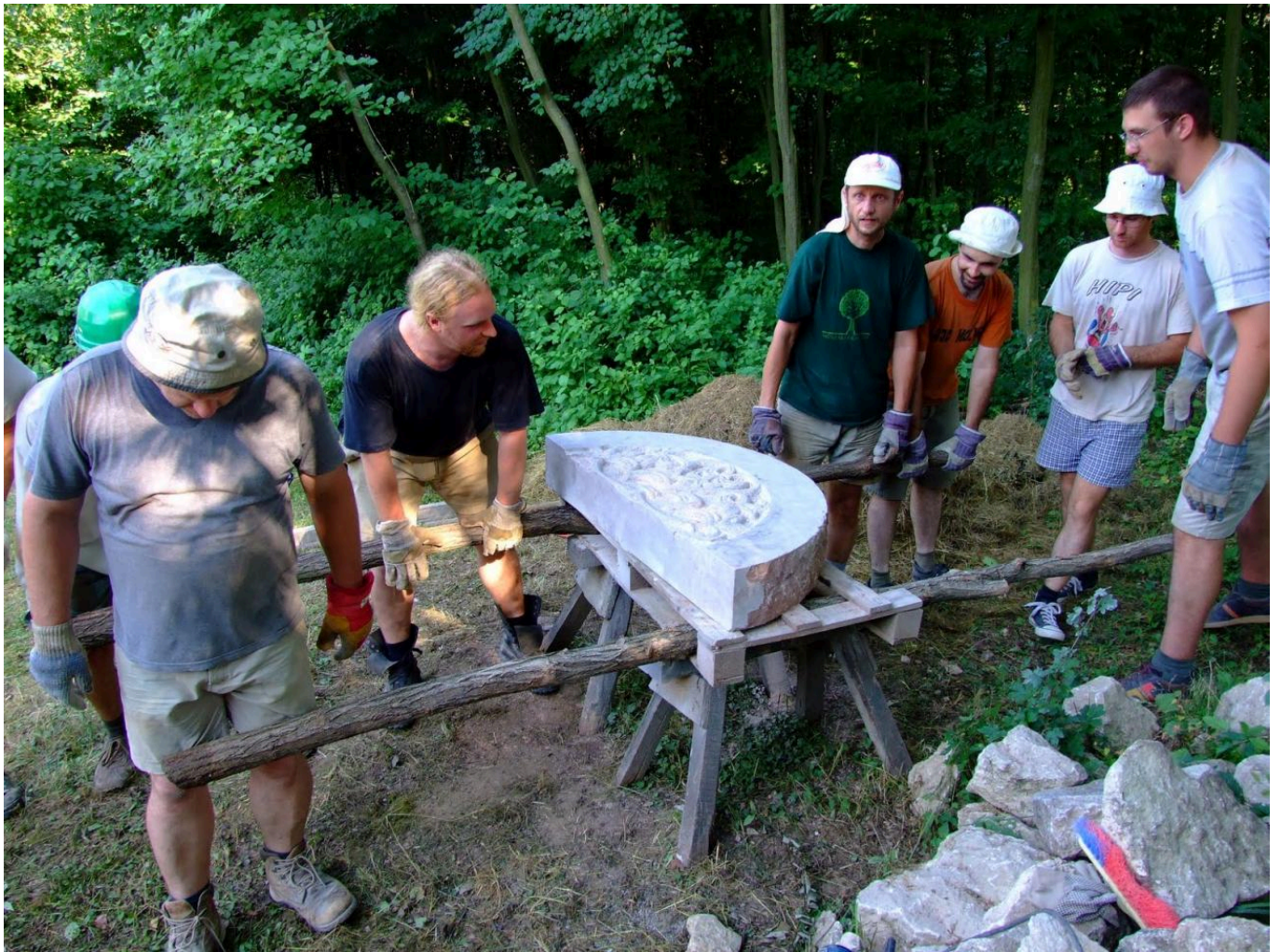
FIG 6C. PICTURES FROM DIFFERENT STAGES OF THE GATE - ARCH RECONSTRUCTION: TRANSPORT OF THE VERY HEAVY HEWN STONES.
