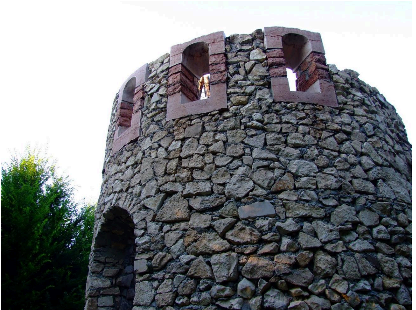
FIG 7D. PICTURES FROM ADVANCED STAGES OF THE RECONSTRUCTION - THE VAULTING STARTS IN LINE WITH THE UPPER LEVEL OF THE WINDOWS.
