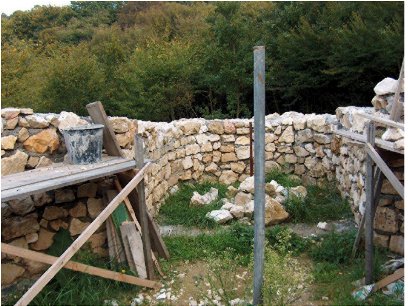
FIG 5B. PICTURES FROM DIFFERENT STAGES OF THE RECONSTRUCTION - WALLING FROM LOW (CA. 1.5 M HIGH) SCAFFOLDING.
