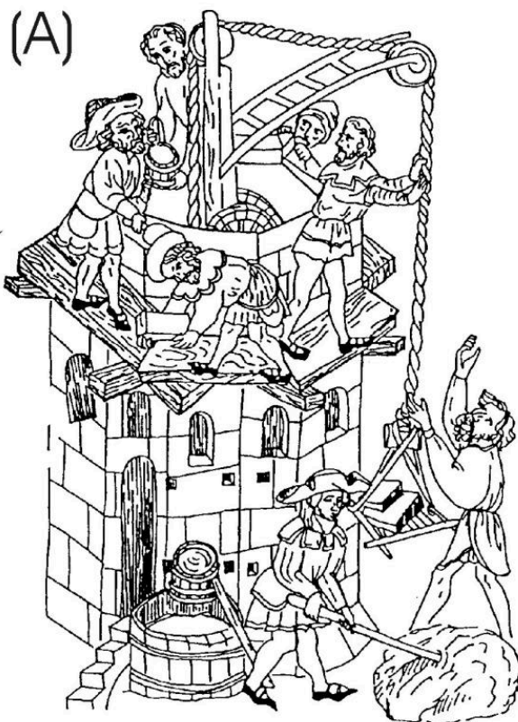
FIG 11. THE MINIATURES SHOW THE PROCESS OF WALL BUILDING USING STONES CUT TO REGULAR SHAPE.
