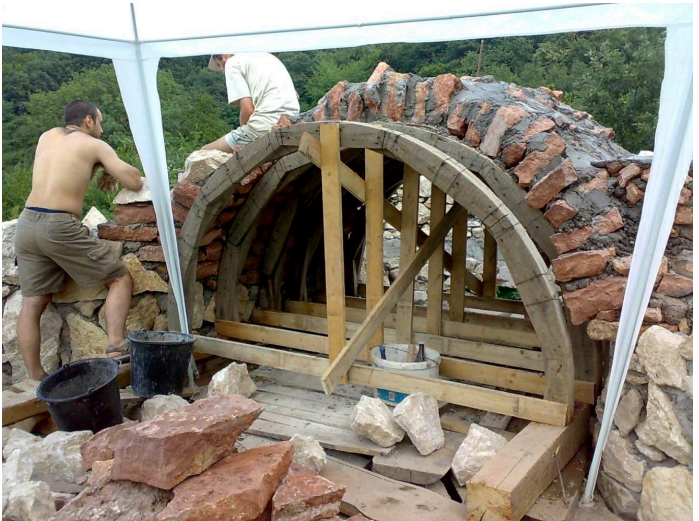
FIG 7B. FURTHER PICTURES FROM ADVANCED STAGES OF THE RECONSTRUCTION - BUILDING OF THE APSE VAULT.
