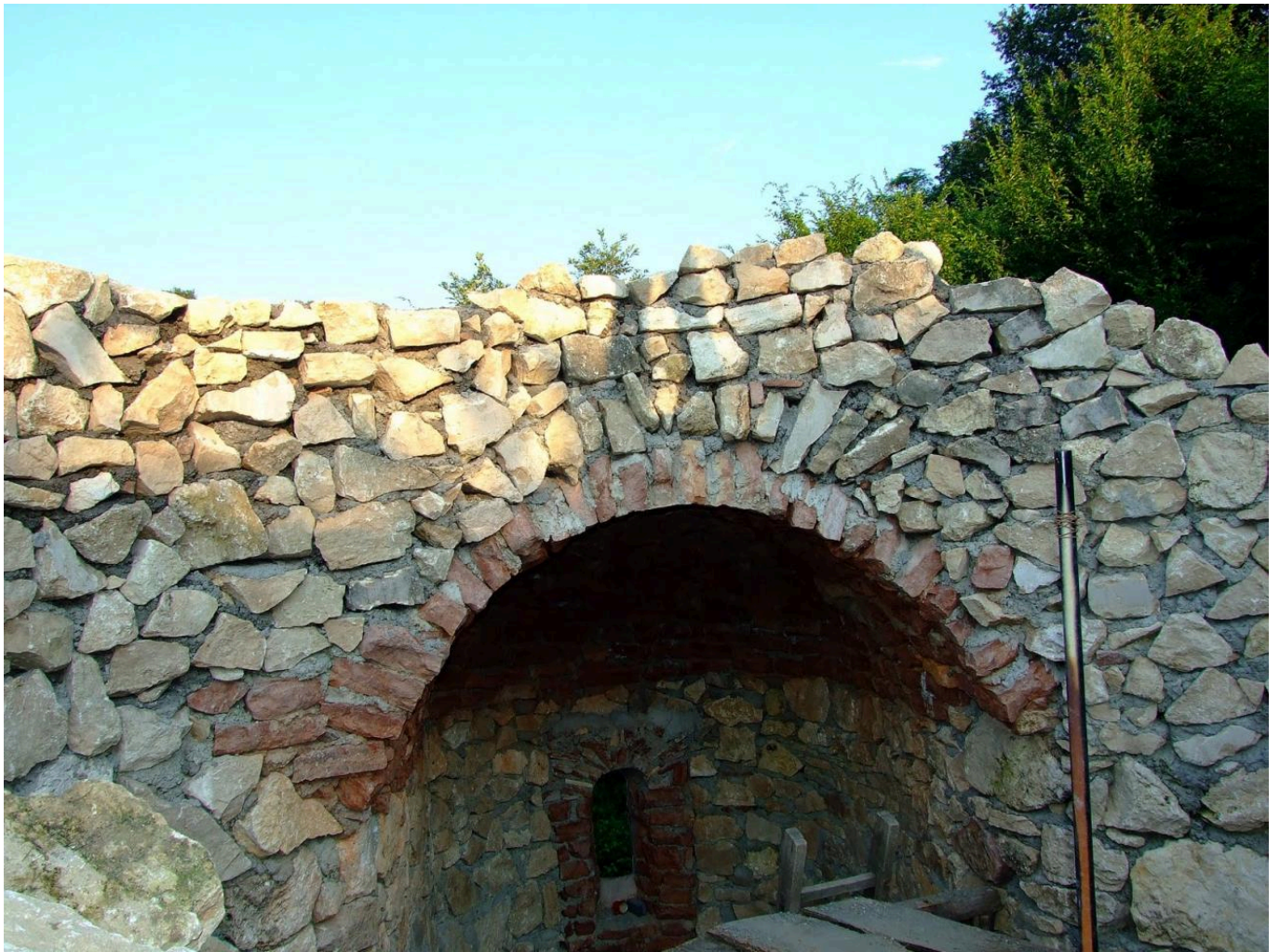
FIG 7C. FURTHER PICTURES FROM ADVANCED STAGES OF THE RECONSTRUCTION - THE VAULTING OF THE APSE IS COVERED BY THE KNEE WALL.
