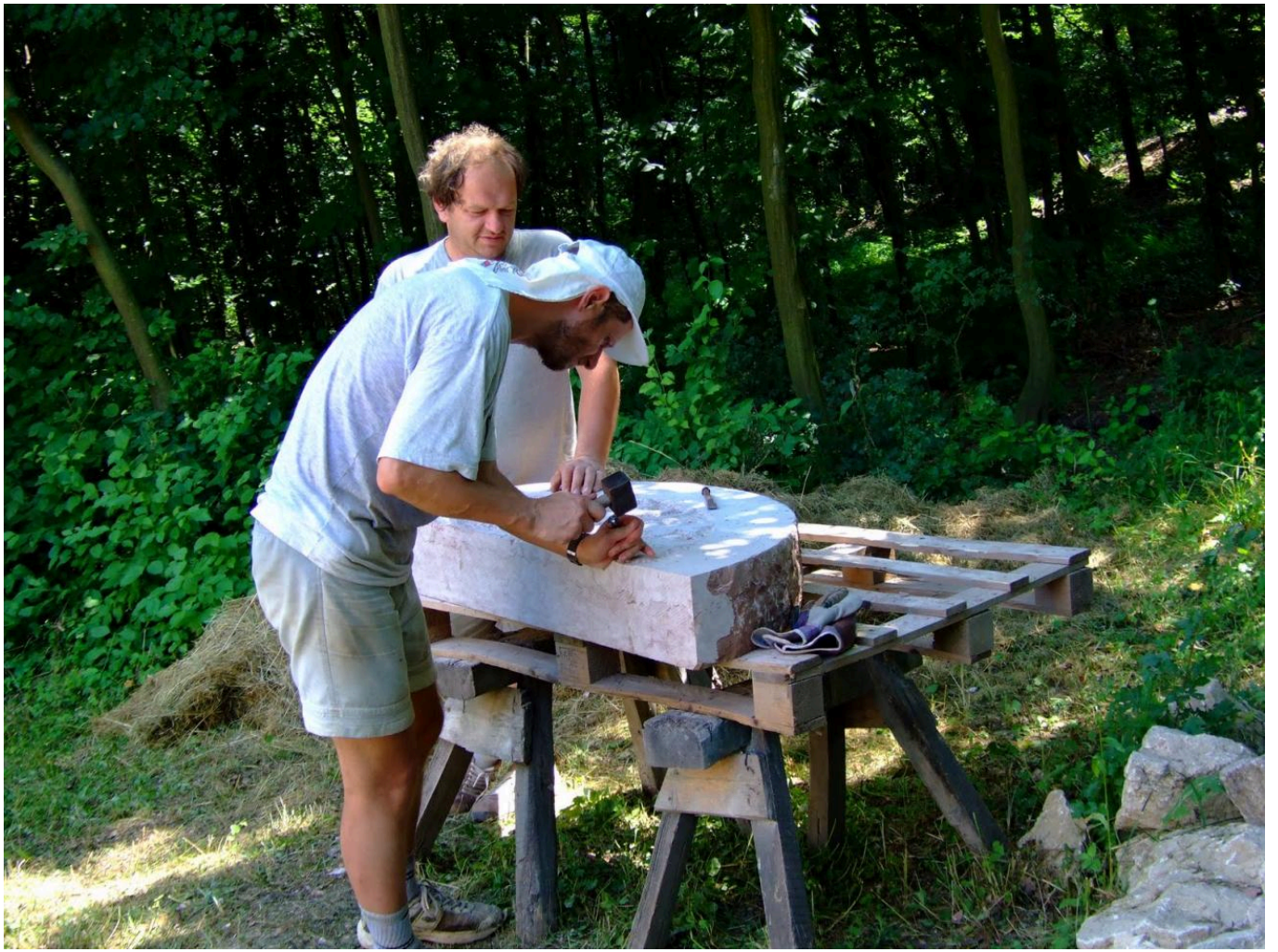
FIG 6B. PICTURES FROM DIFFERENT STAGES OF THE GATE - ARCH RECONSTRUCTION: CUTTING OF THE RELIEF.
