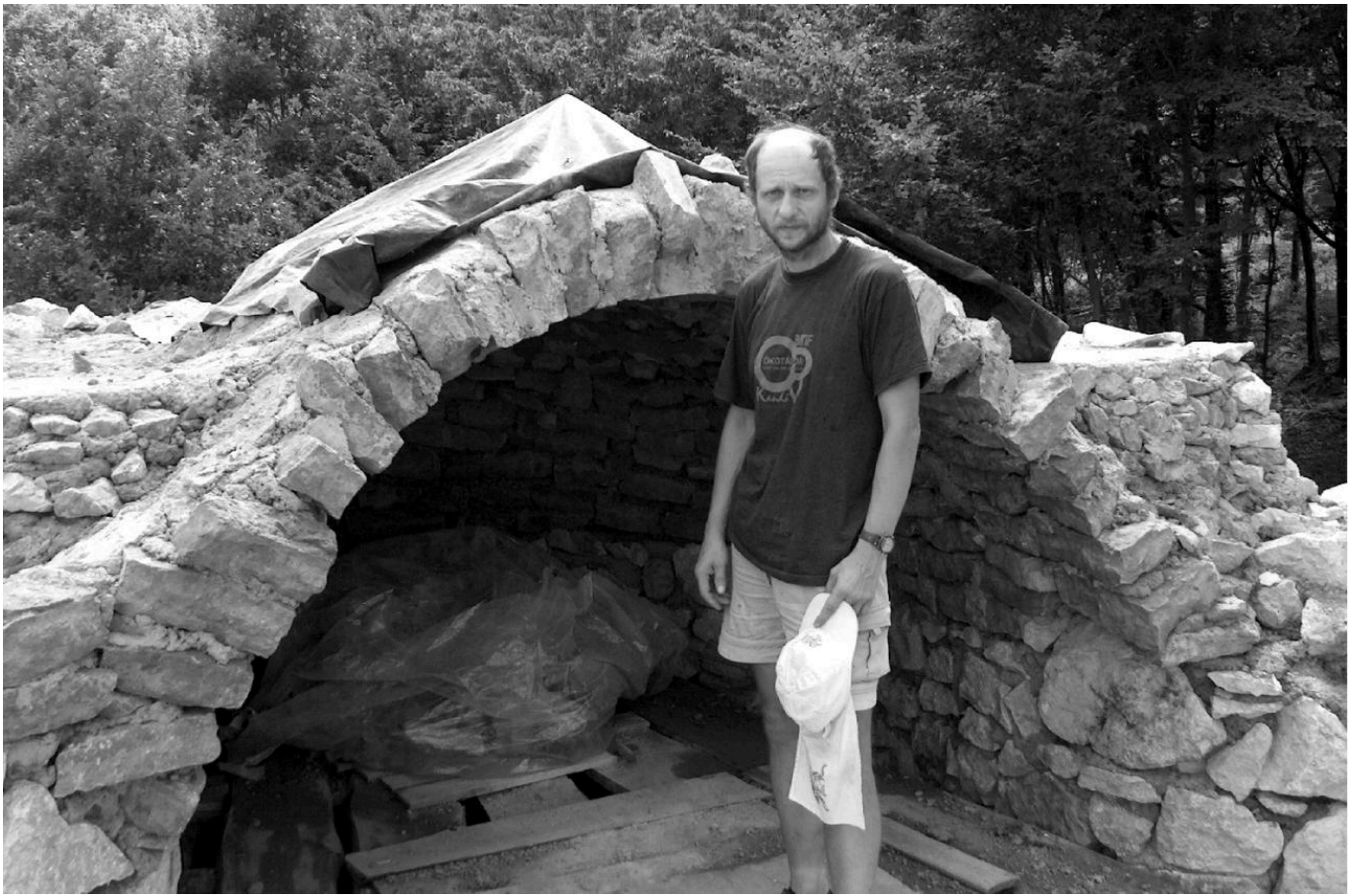
FIG 17B. THE ERECTION OF THE APSE VAULTING - THE APSE VOLT BUILDING CARRIED OUT FROM THE EXISTING WALL.
