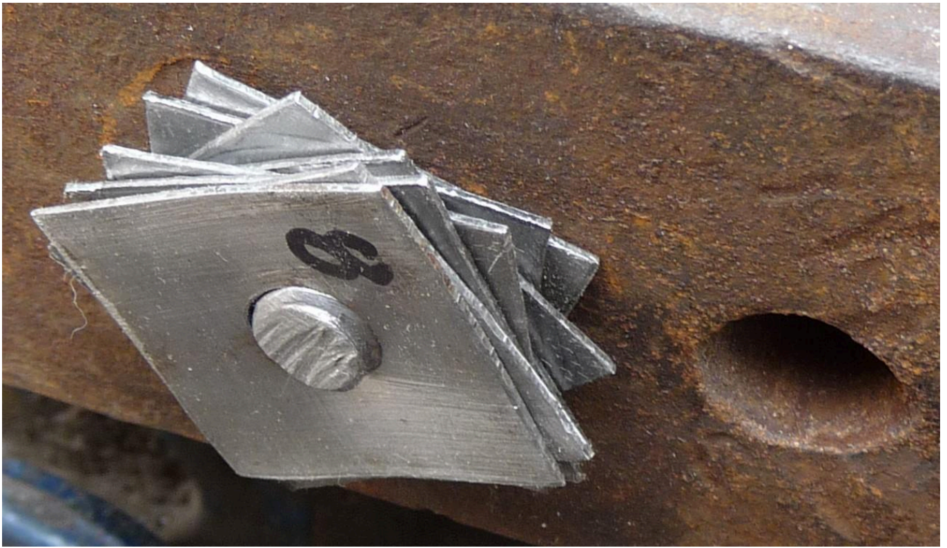
FIG 28. SHOWS SEVEN PIECES OF IRON TAPPED AND SCREWED ONTO THE BOLT TO FORM A NUT. PHOTO BY DAVID SIM
