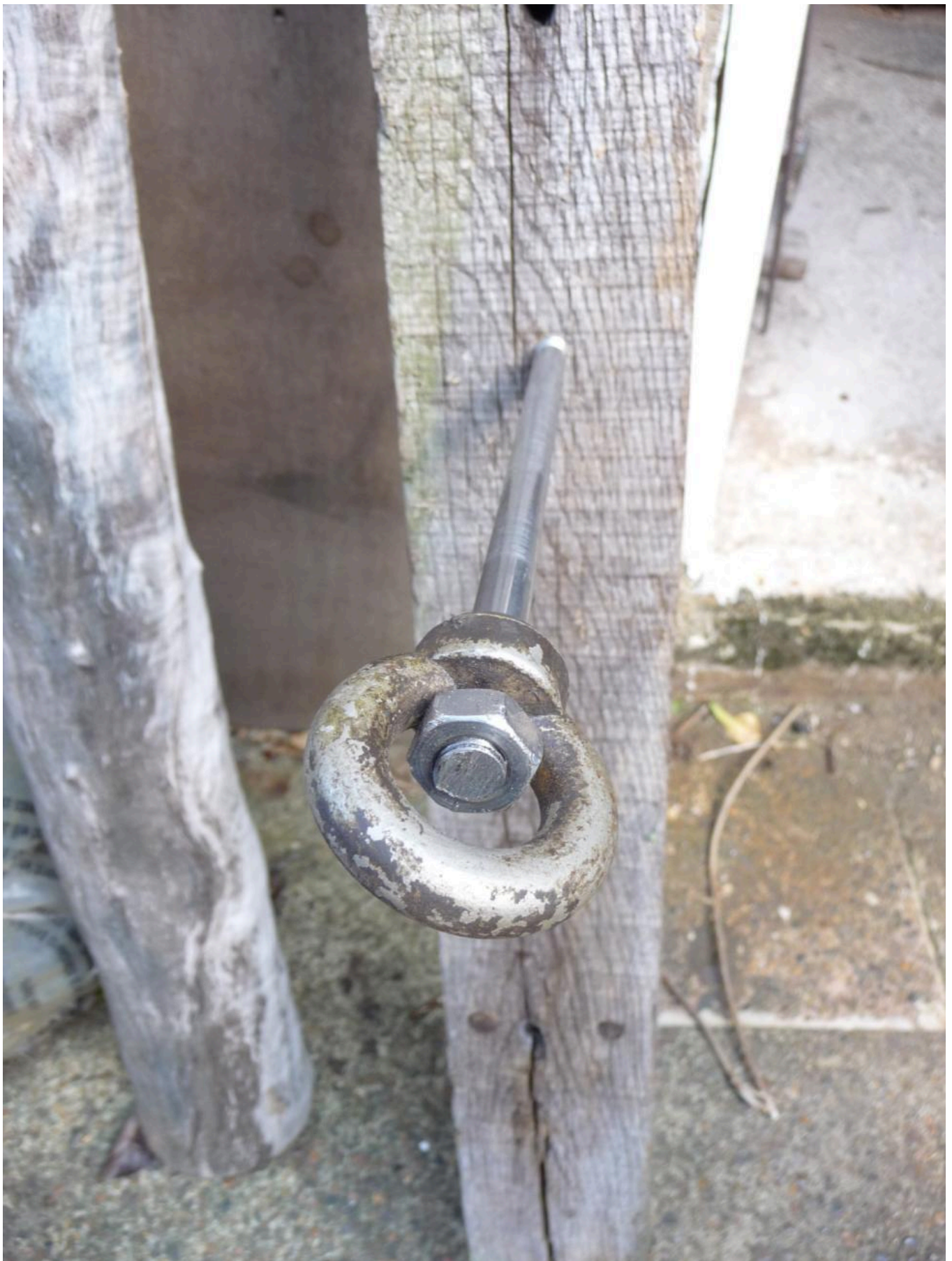
FIG 30. THREAD WITH EYE BOLT ATTACHED. PHOTO BY DAVID SIM.
