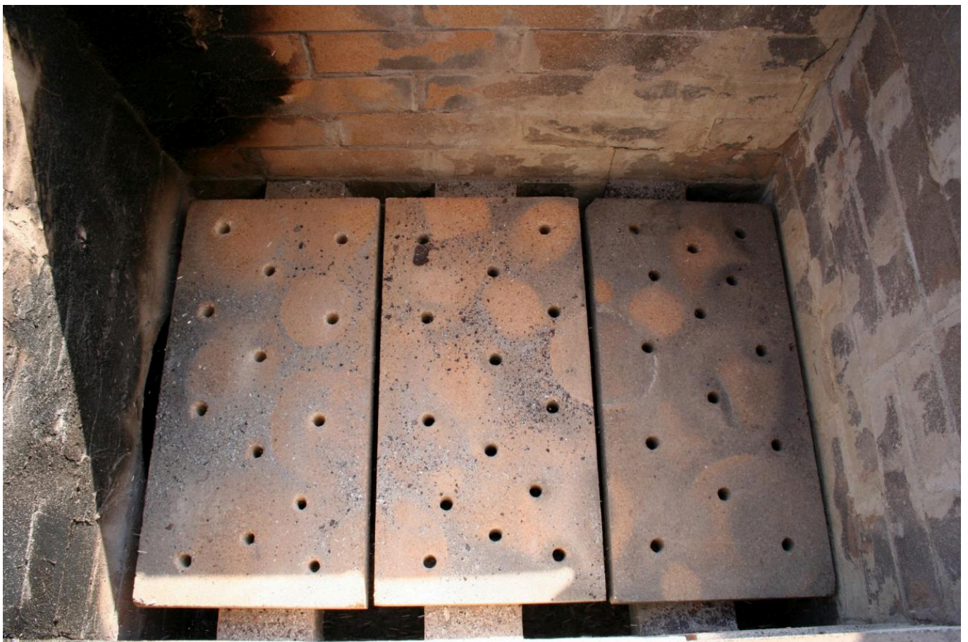
FIG 2. THE INTERIOR OF THE UPDRAFT WOOD-FIRING KILN WITH THE LATERAL OPEN SIDES. PHOTO BY GEORGIA KORDATZAKI
